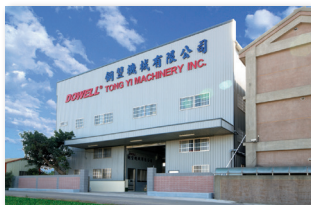
銅翌二廠 DOWELL-Second Factory
