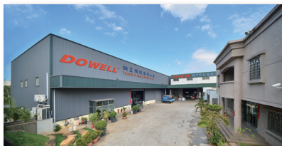
銅翌一廠 DOWELL-First Factory
